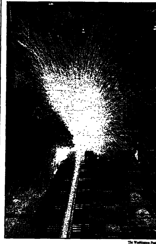
Steel being rolled into rail at a Wheeling-Pittsburgh mill.
